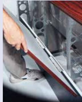
Permanent front panels can be installed if easy access to the equipment and utilities from the customer side is not required.
