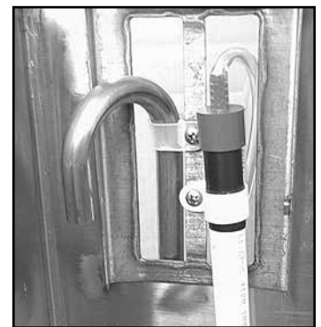
Stainless Water Inlet Tube and Low-Level Sensor Pick-Up Tube (Cover Removed)
