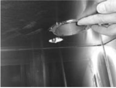
9. Air cooled towers that mount directly above the keg cooler include a top hat sleeve. Mount the sleeve from inside the cooler upward with the four #10x1/2" phillips pan head s/s screws provided.
