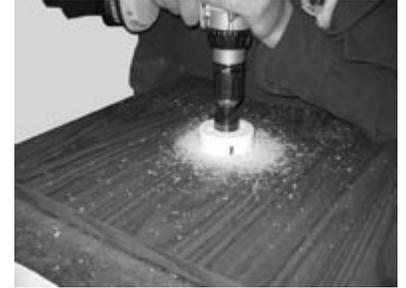
7. Enlarge the beer line hole using a 1/4" drill bit and then finish at 3-1/4" using an appropriately sized hole saw.
