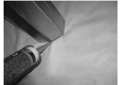
14. Apply a bead of silicone sealant around the perimeter of the column. Use your index finger to smooth out the bead.
