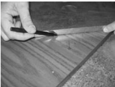
4. Using a straight edge and the four column stiffener mounting holes, mark the center of the beer line hole.
