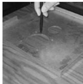
3. Position the drain pan base plate in the desired location and mark all holes.
