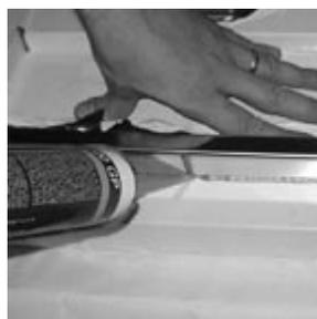
17. Apply a bead of silicone sealant around the perimeter of the drain pan. Use your index finger to smooth out the bead.
