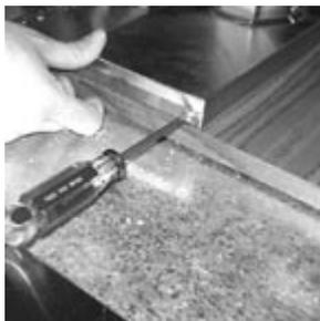
13. Secure the drain pan to the base plate with the four #10-32 phillips pan head s/s machine screws provided (will be brass screws for brass towers).
