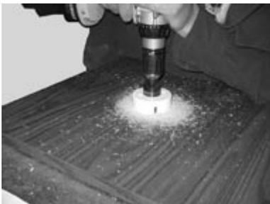
5. Enlarge the beer line hole(s) using a 1/4" drill bit and then finish at 3-1/4" using an appropriately sized hole saw.
