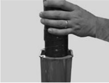
9. If the tower is air cooled, install the insulation provided into the column stiffener.
