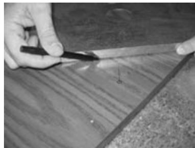
2. Using a straight edge and the four column stiffener mounting holes, mark the center of the beer line hole(s).
