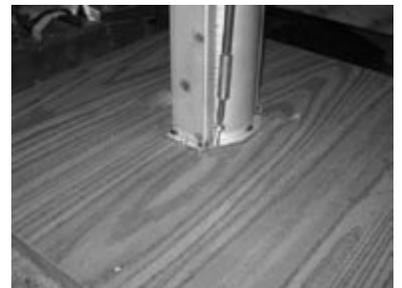
8. Mount the column skin with the four #14x1-1/4" phillips pan head sheet metal screws provided, or use your own screws if more appropriate for your installation.
