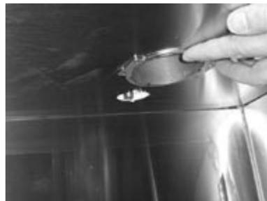
7. Air cooled towers that mount directly above the keg cooler include a top hat sleeve. Mount the sleeve from inside the cooler upward with the four #10x1/2" phillips pan head s/s screws provided.
