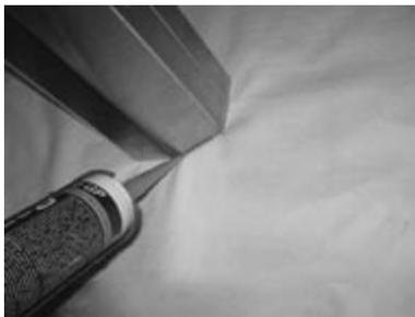
13. Apply a bead of silicone sealant around the perimeter of the column. Use your index finger to smooth out the bead.
