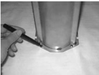
1. Place the column stiffener in the desired location and mark the four mounting holes. For remote cooled towers use the paper template located on the back of this sheet. For two column tee towers, use metal template supplied.
