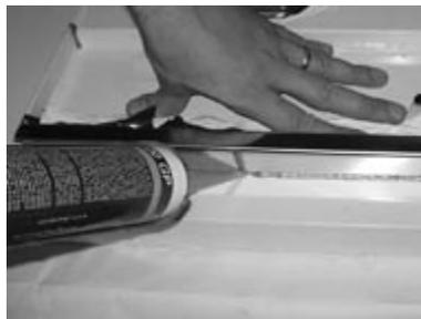
16. Apply a bead of silicone sealant around the perimeter of the drain pan. Use your index finger to smooth out the bead.
