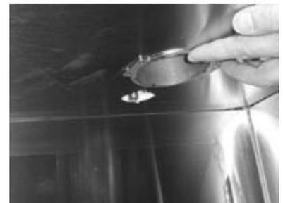
8. Air cooled towers that mount directly above the keg cooler include a top hat sleeve. Mount the sleeve from inside the cooler upward with the four #10x1/2" phillips pan head s/s screws provided.
