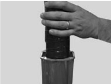
12. If the tower is air cooled, install the insulation provided into the column stiffener.
