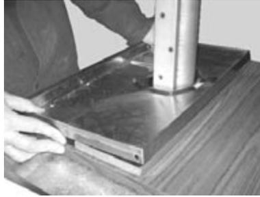
10. Place the drain pan over the column stiffener and base plate.
