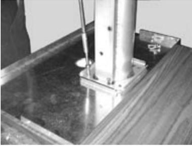
9. Mount the column stiffener with the four #14x1-1/4" phillips pan head sheet metal screws, provided, or use your own screws if more appropriate for your installation.
