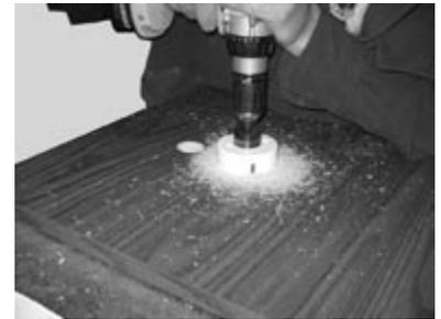
5. Drill the beer line hole(s) and drain hole to 1/4". Finish the drain hole at 1-1/2", and the beer line hole at 3-1/4" using an appropriately sized hole saw.
