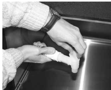
Drain valve operation detail
